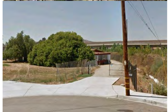
Site 33: Underutilized residential parcel with single-family home built in 1958. Site is adjacent to another underutilized site with single-family home built in 1954
