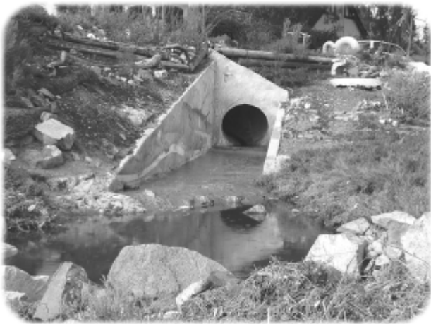
A storm drain outlet that empties directly into a local stream.
