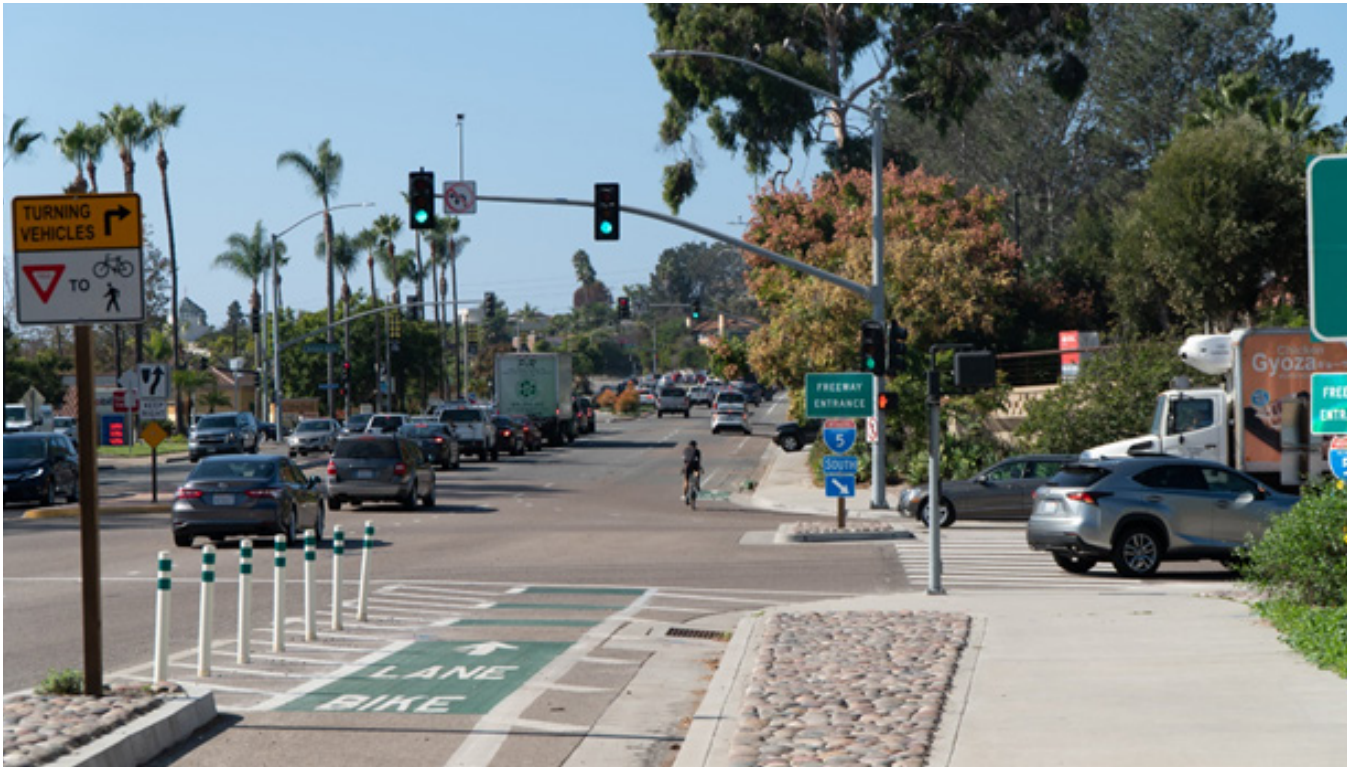
Bike Lane Conflict Paint on approach Leg of local street at freeway on-/off-ramp
