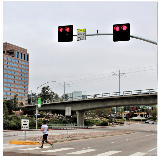
San Diego River Trail hybrid beacon crossing in the City of San Diego
