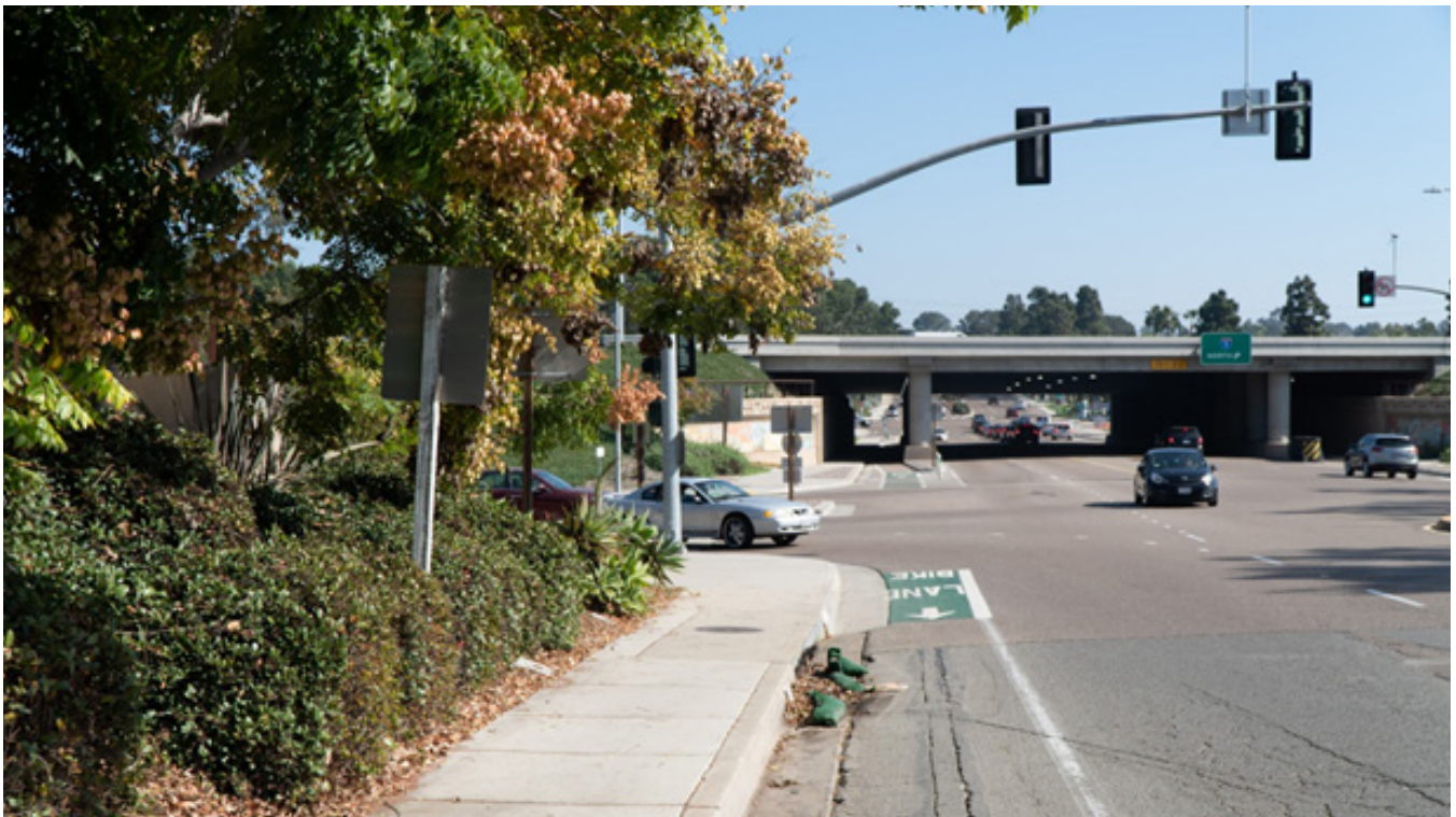
Bike Lane Conflict Paint on departure leg of local street at freeway on-/off-ramp
