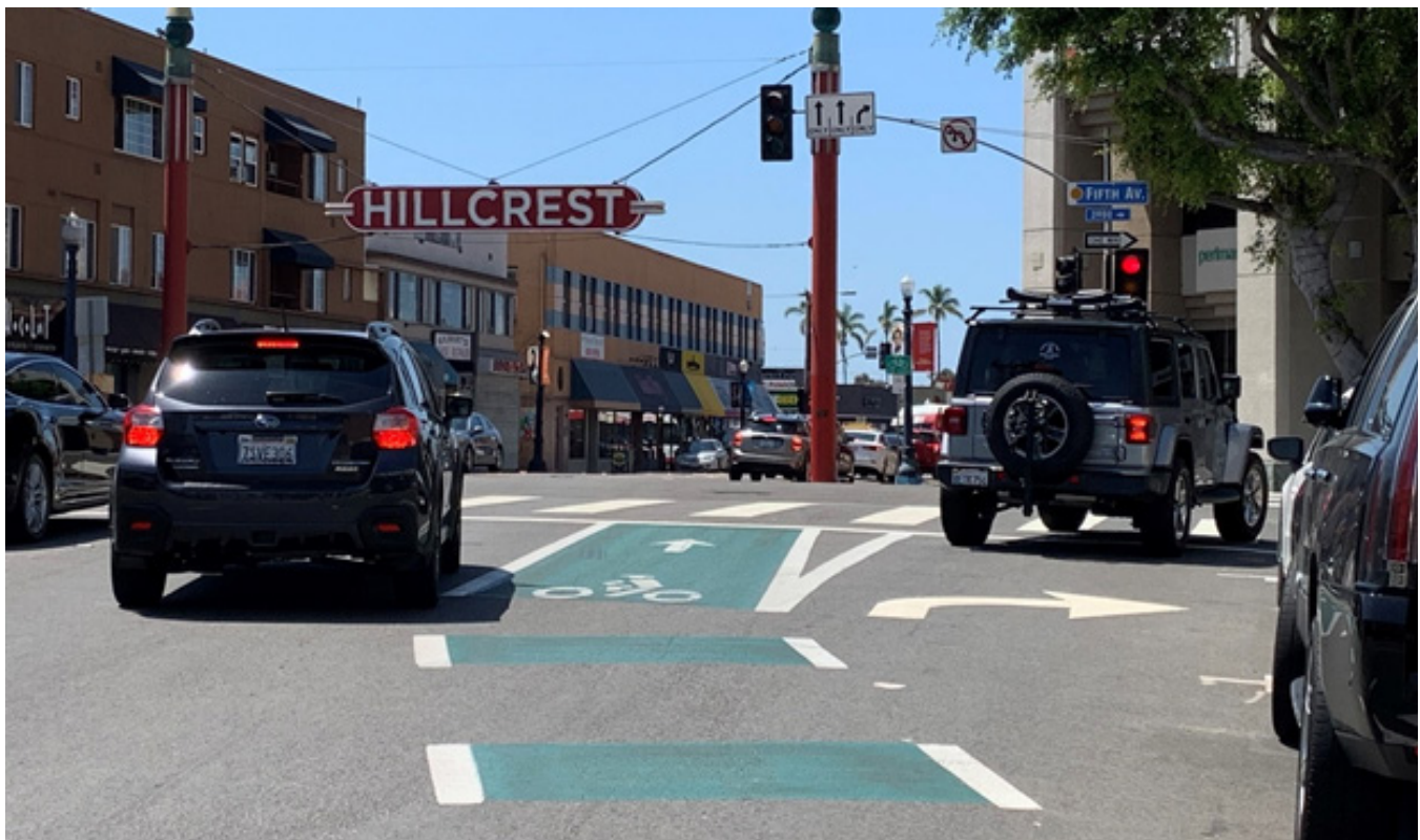
Dashed conflict paint used to emphasize the bike lane at a right-turn only lane
