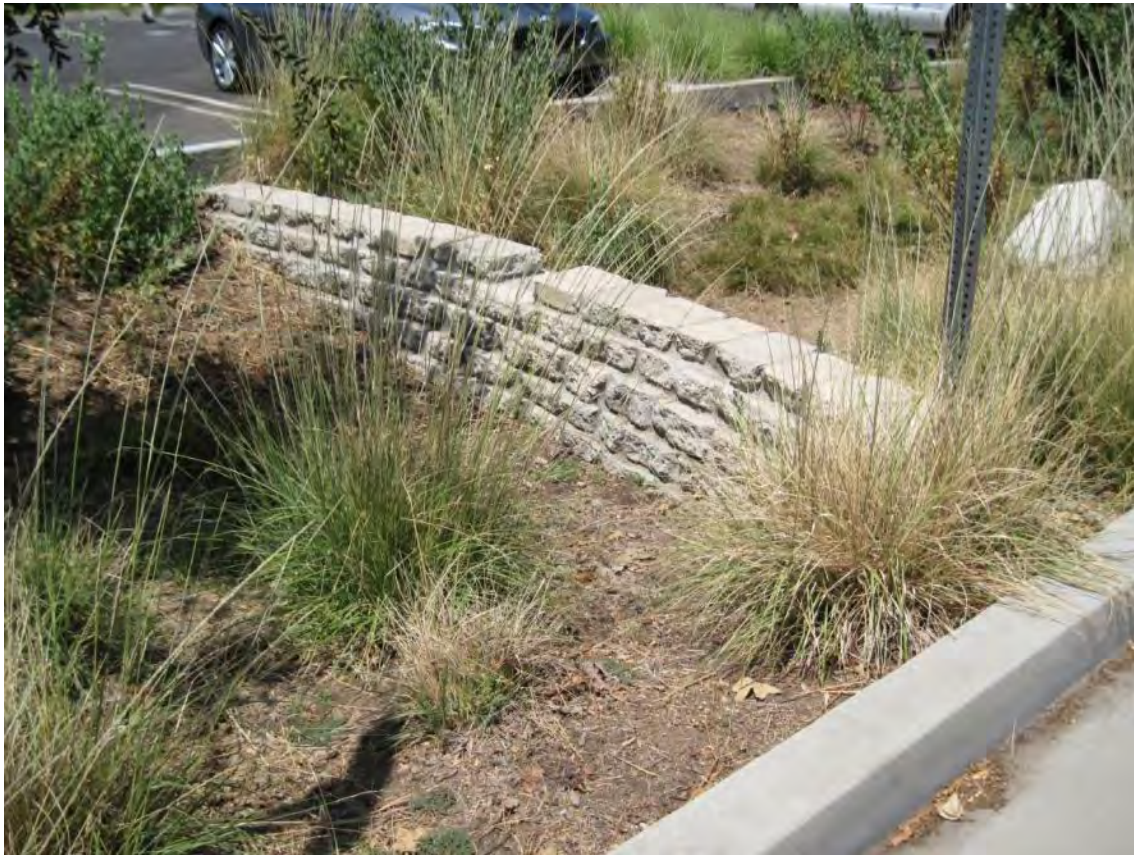
Figure A.2-7. Bioretention swale with a check dam.
