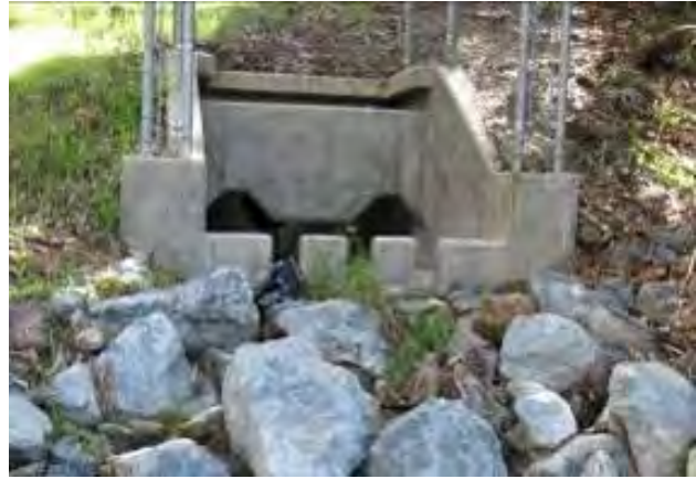
Figure A.11-3. Constructed concrete energy dissipater.
