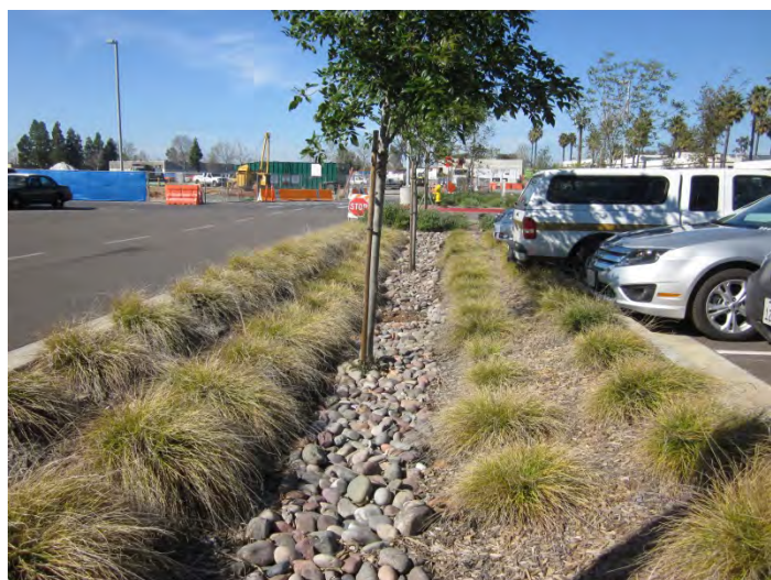
Location: County Operations Center, San Diego, California.
