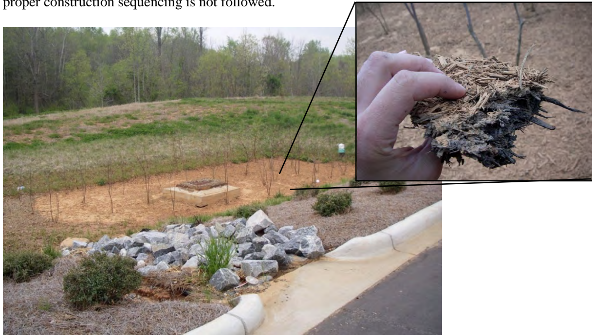
Figure 4-1. Example of a bioretention area installed before permanent site stabilization, with the inset photo showing the clay layer clogging the mulch surface.
