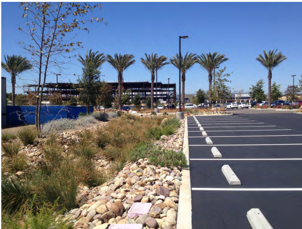
Figure 4-29. Roads and parking lots are graded towards bioretention areas that treat runoff near its source.
