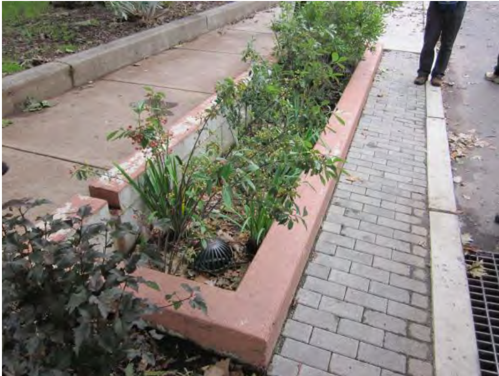
Figure 3-31. Roadside flow-through planter.
