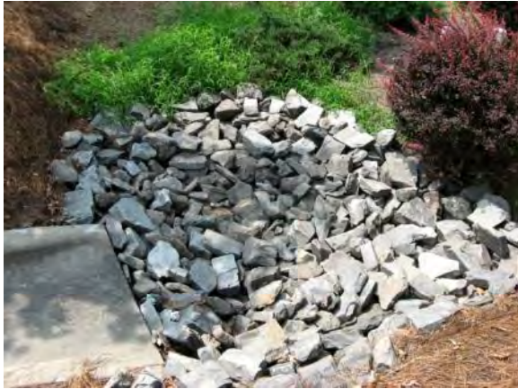
Figure A.11-2. Rock forebay.
