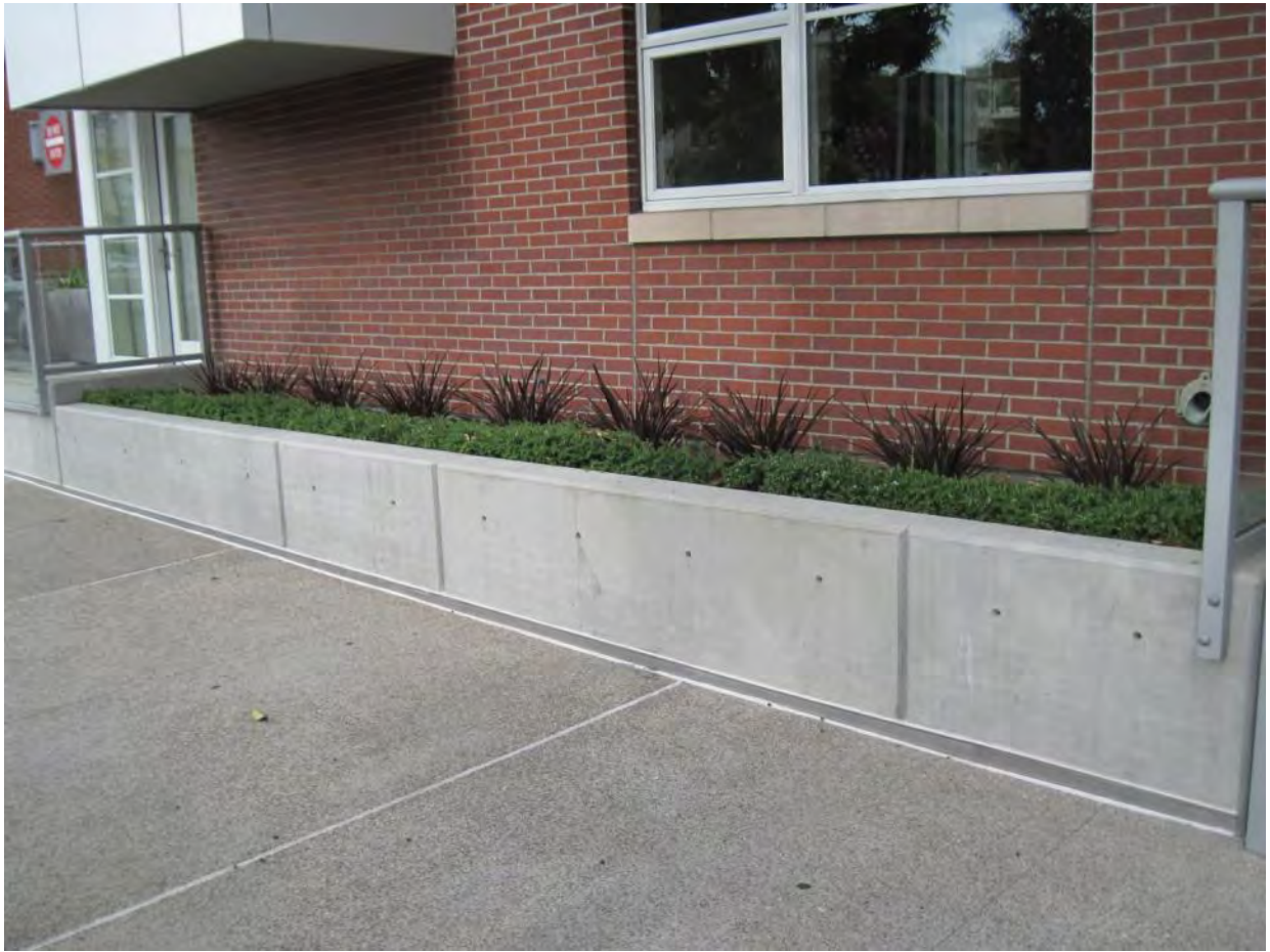
Figure A.5-1. Flow-through planter.
