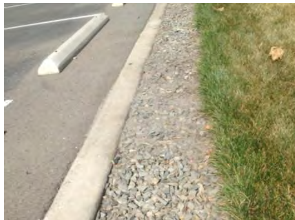
Figure A.11-5. Gravel flow spreader.
