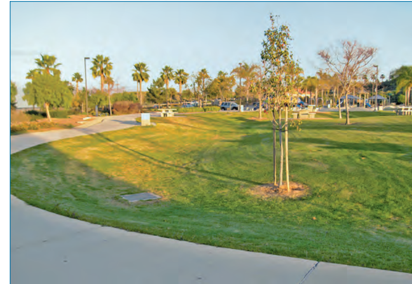
A vegetated swale conveys and treats runoff from a public park. Proper design, maintenance of dense vegetation, and accurate fine grading ensure optimum treatment and minimize the risks of erosion or standing water.
