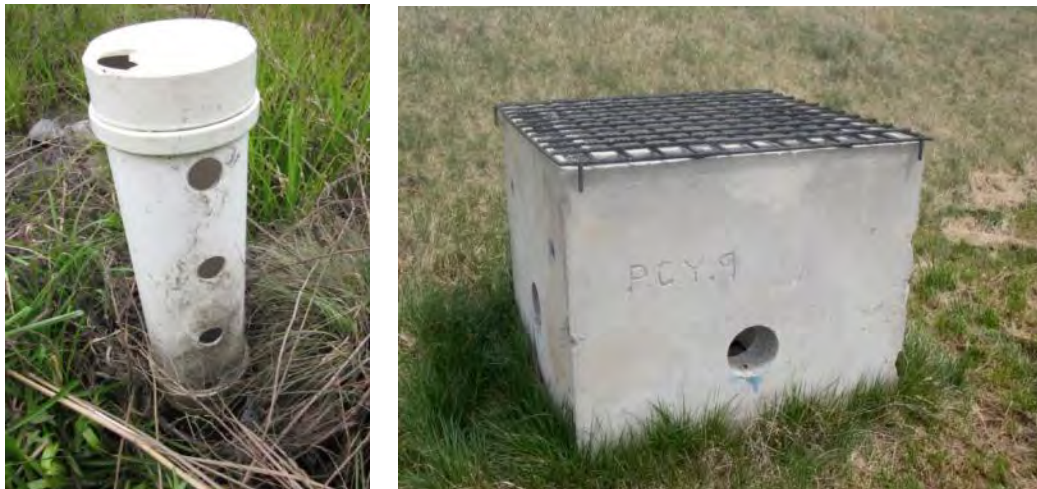
Figure A.1-14. Bioretention outlet structures designed for peak flow mitigation.
