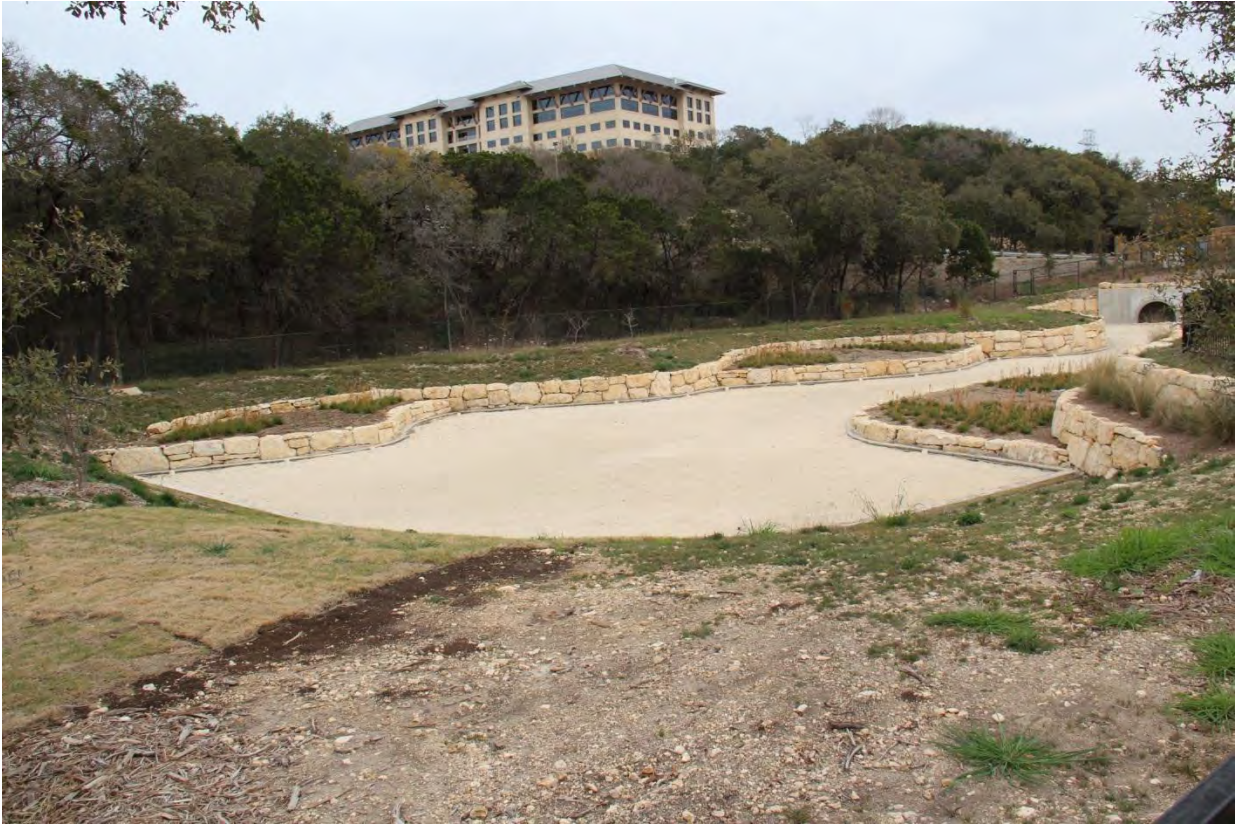
Figure A.7-1. Surface sand filter treats parking lot runoff.
