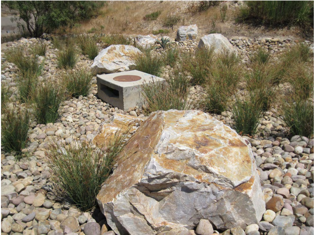
Figure 4-31. Bioretention areas with raised outlet structures are distributed throughout the site to transform traditional landscaped areas into stormwater IMPs.
