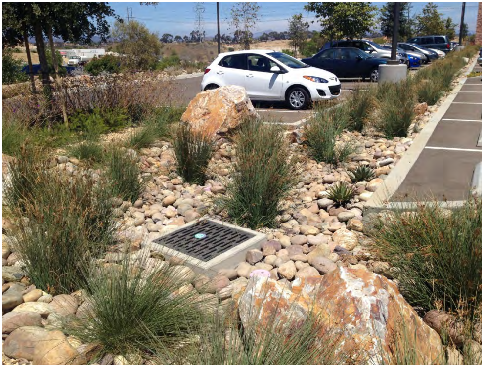
Figure 4-28. Bioretention swales with raised outlet structures capture, convey, and filter parking lot runoff through a soil media layer.
