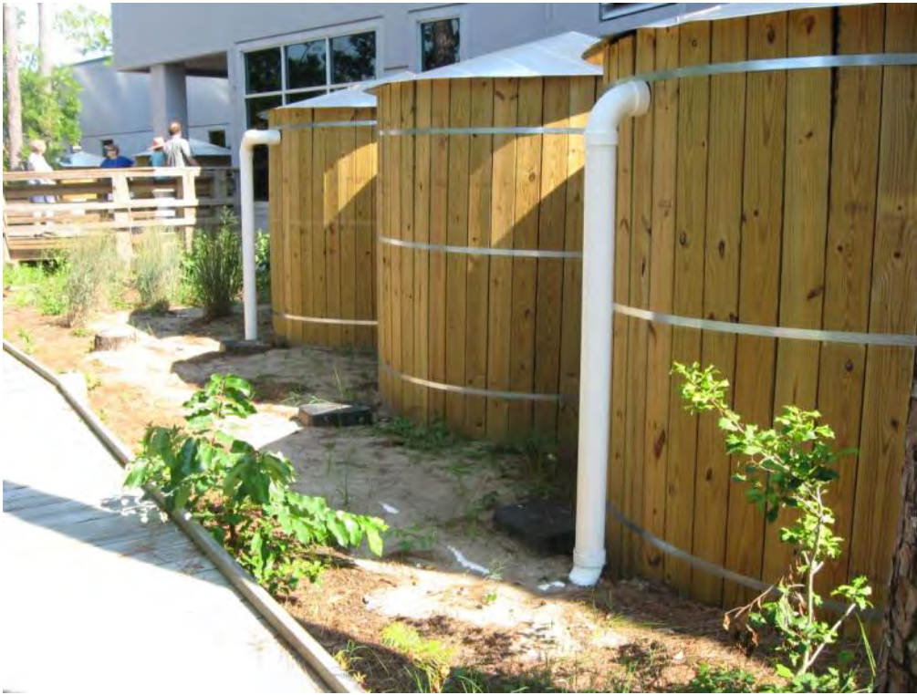
Figure 3-40. Wood wrapped cistern.
