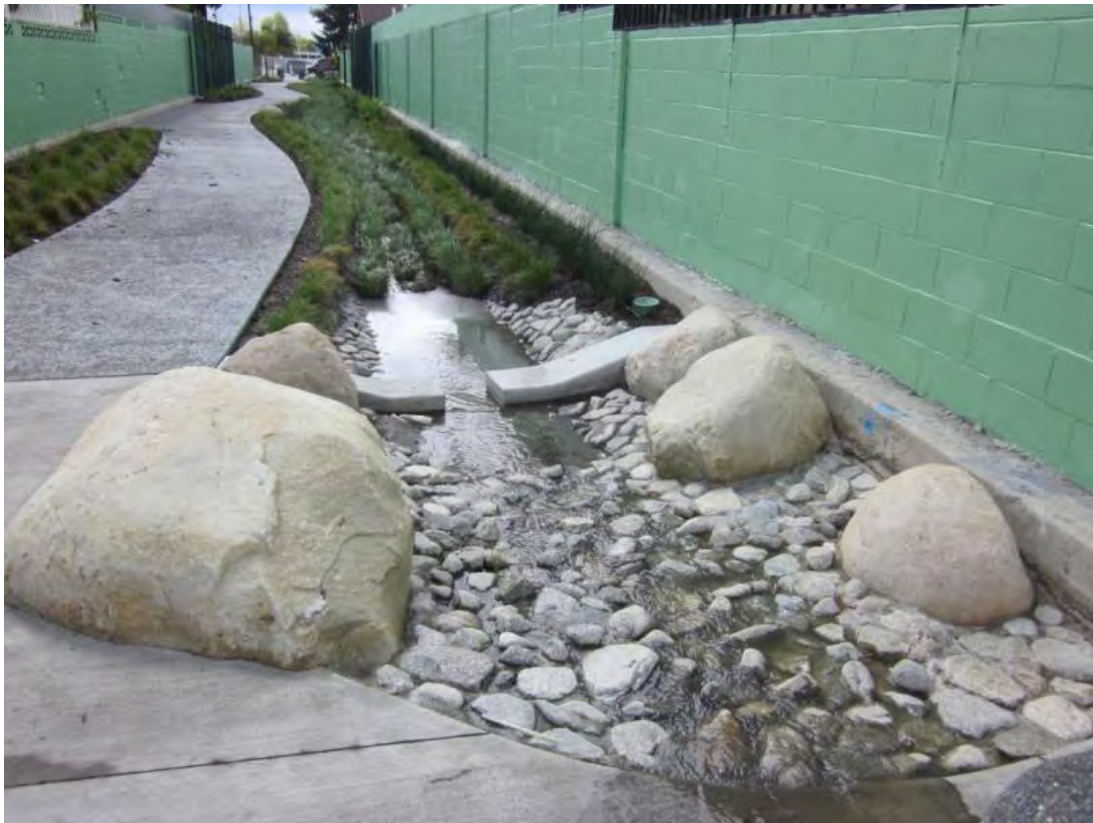
Figure A.1-9. Inlet and pretreatment provided by mortared cobble forebay and energy dissipater.
