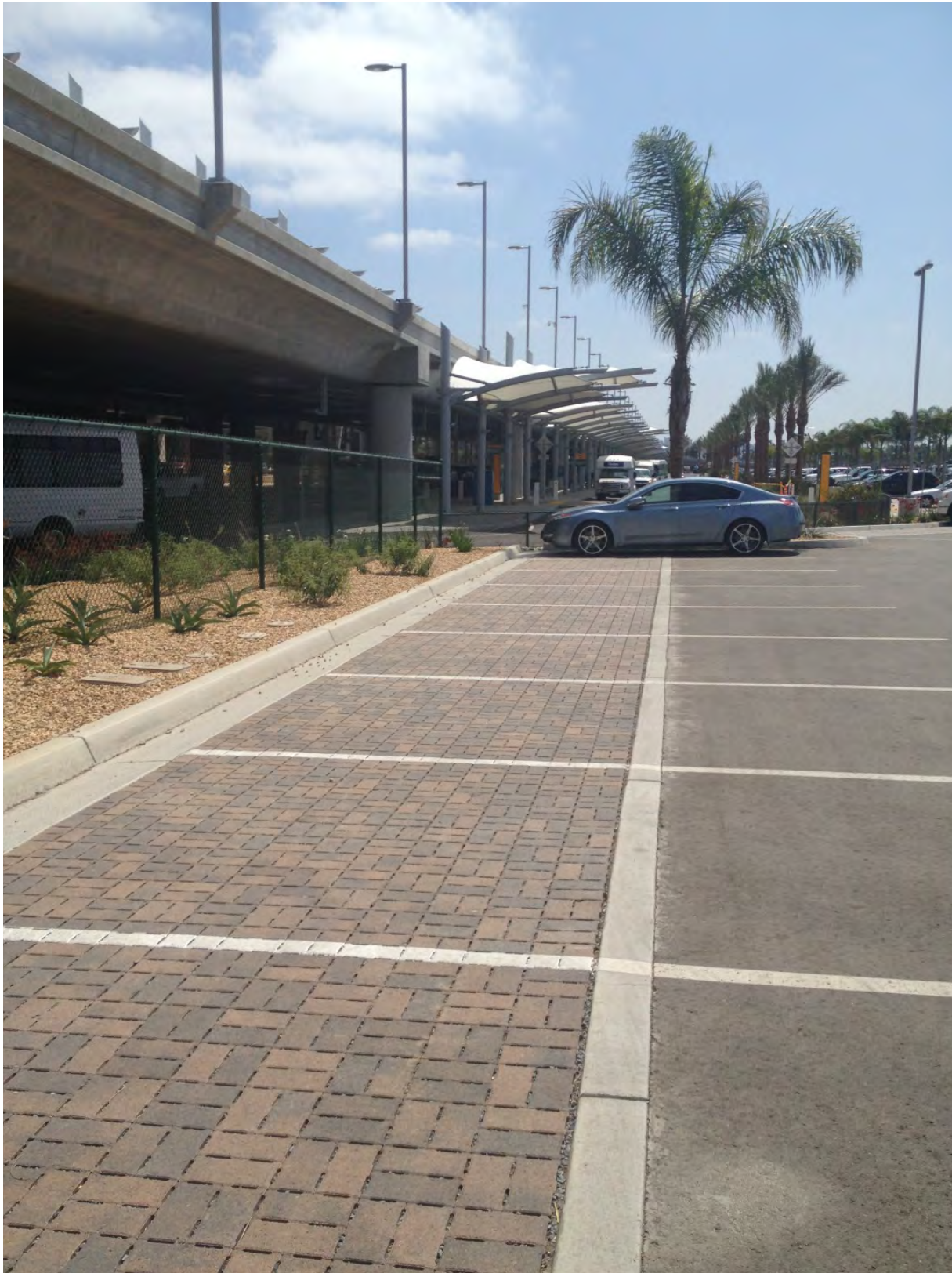
Figure 4-24. A concrete transition strip was used to delineate the permeable surface and provide edge restraints for the pavers.
