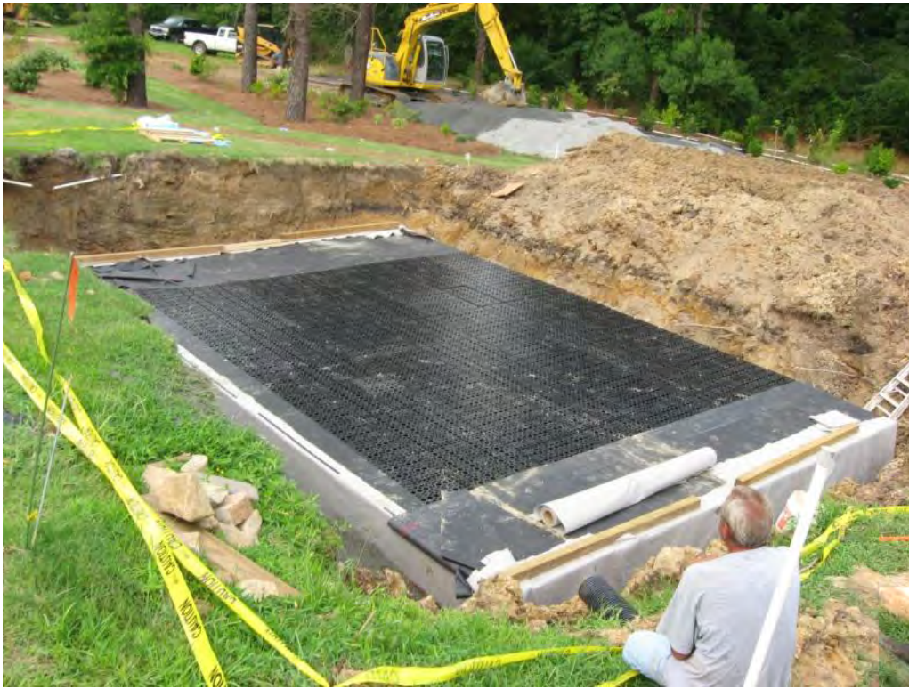
Figure 3-42. Below-ground cistern.
