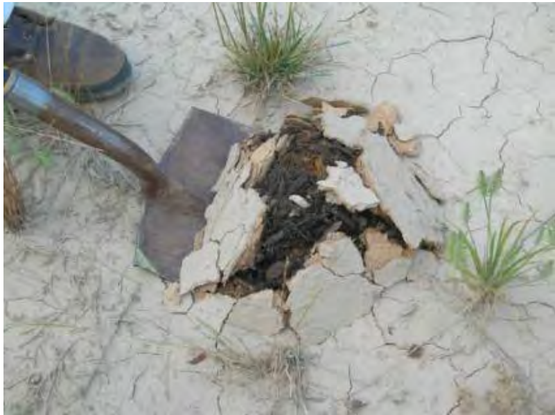
Figure 4-6. Bioretention area clogged with sediment.
