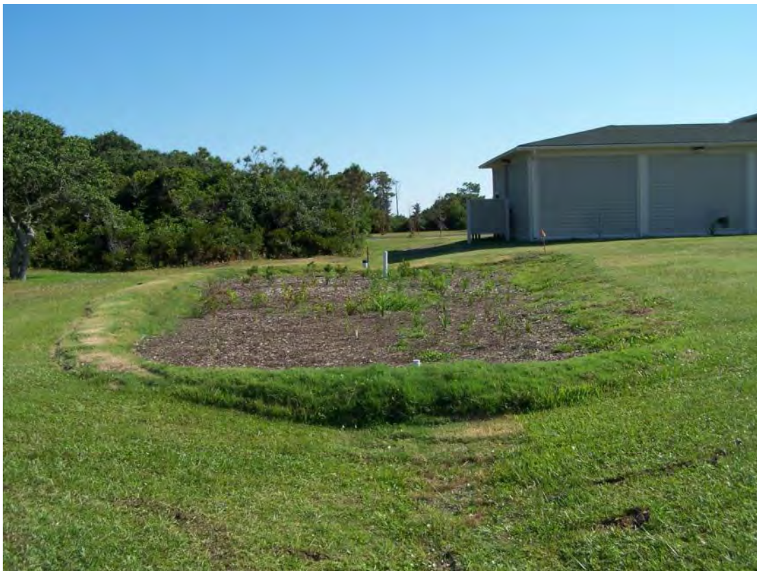
Figure A.1-13. Flow spreaders (illustrated as a stabilized earthen berm in this photograph) can be used to regulate ponding depths in small, online bioretention areas.
