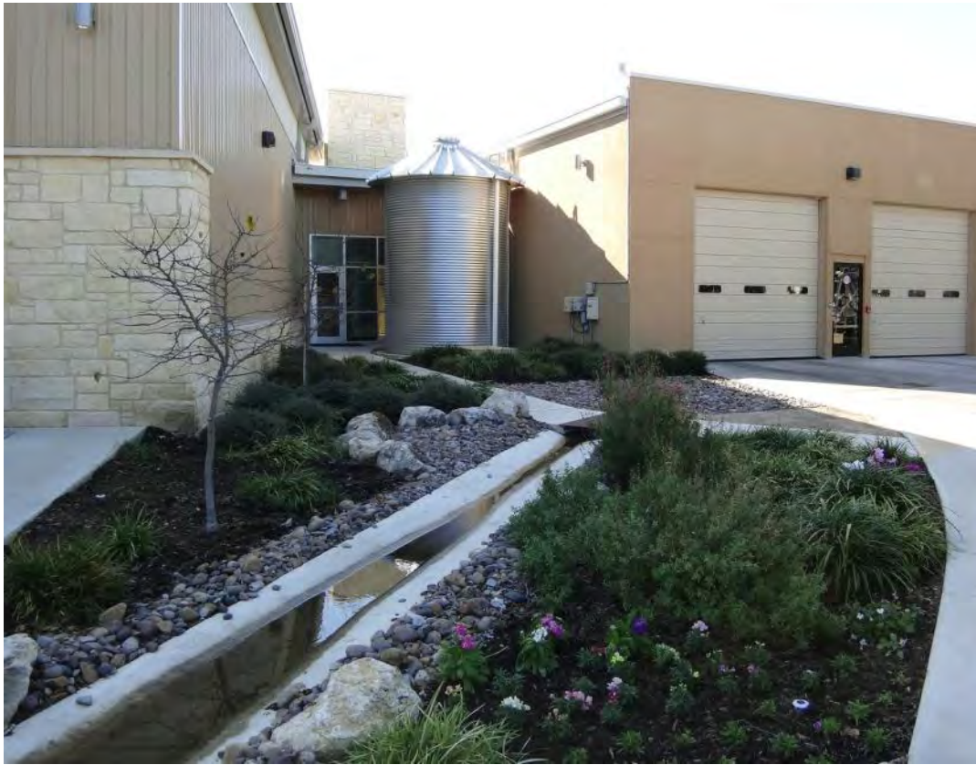
Figure A.8-1. Corrugated metal cistern.
