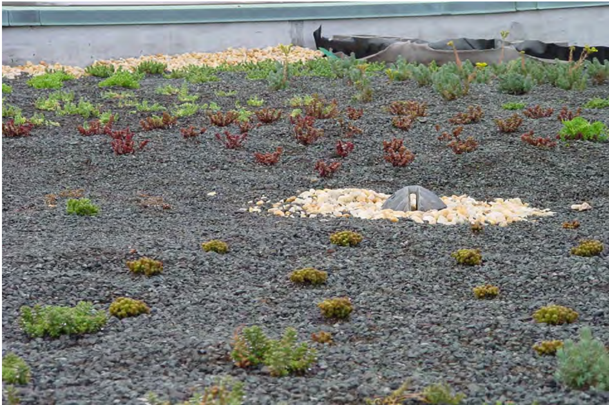
Figure 4-10. No plant zone for a green roof.
