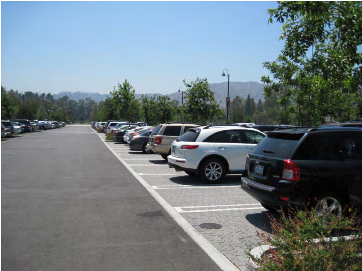
Figure A.3-10. Concrete transition strip between PICP and standard asphalt.
