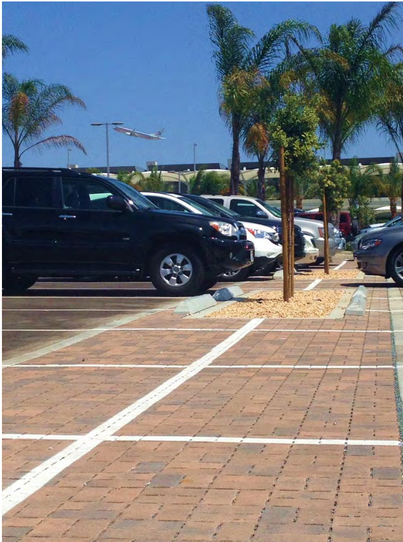
Figure 4-20. Permeable pavement in the Terminal 2 parking lot.
