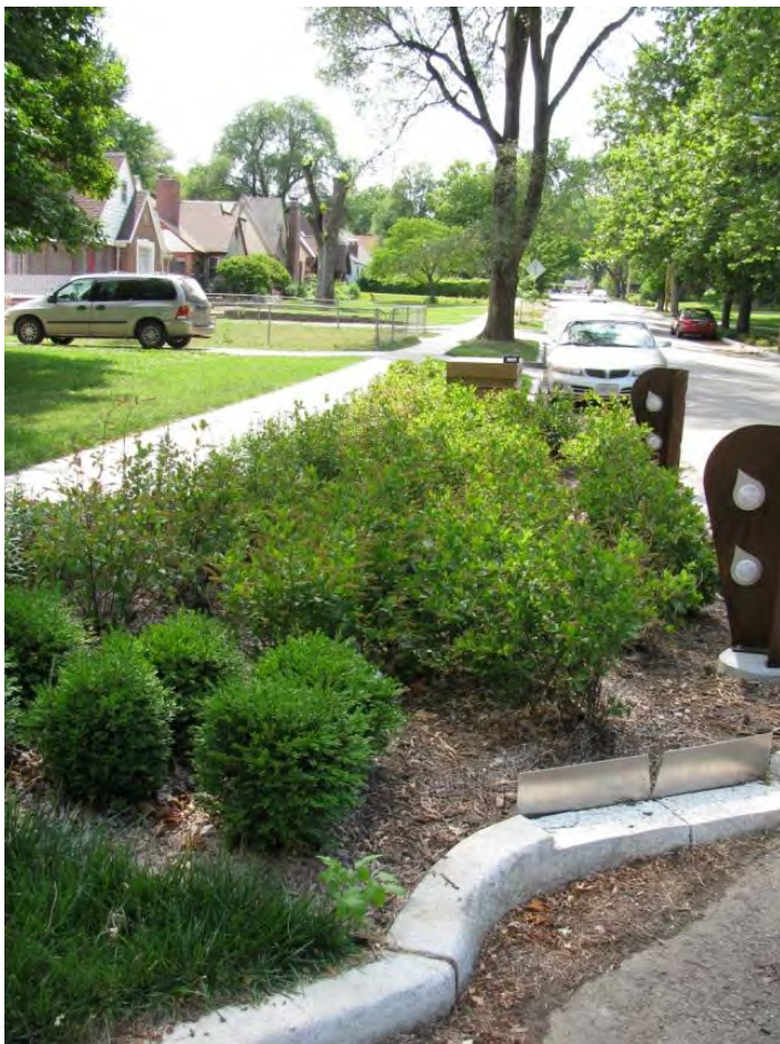
Figure 4-14. Outlet of a roadside bioretention bumpout equipped with a V-notch weir for flow monitoring.
