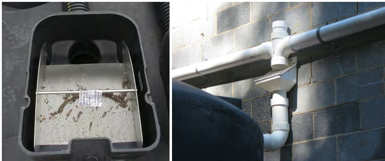
Figure 4-11. Self-cleaning inlet filters.
