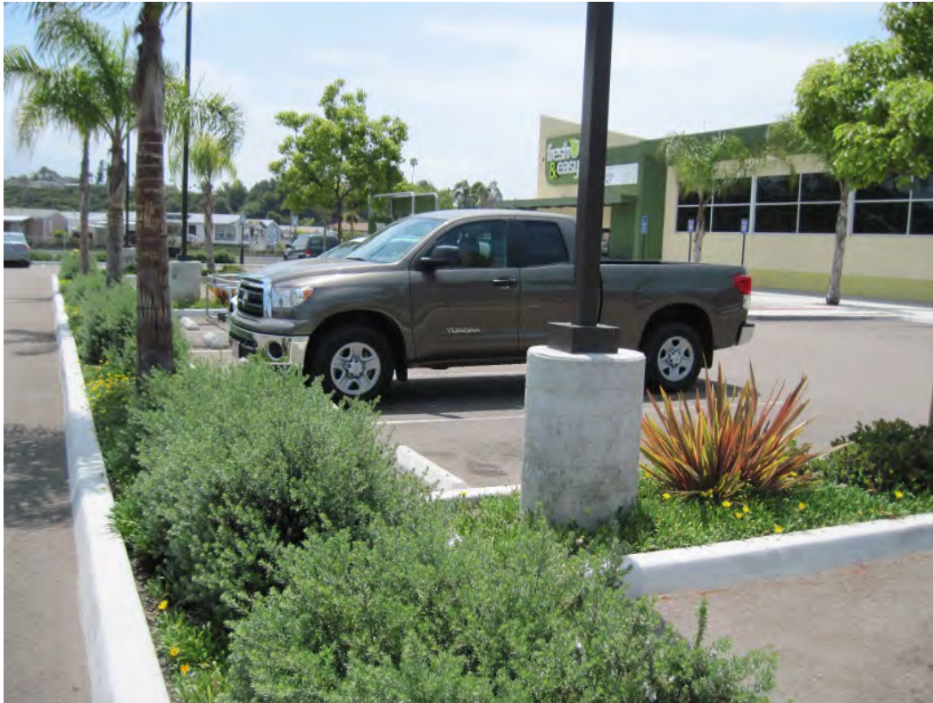
Figure 3-19. Parking lot bioretention swales.
