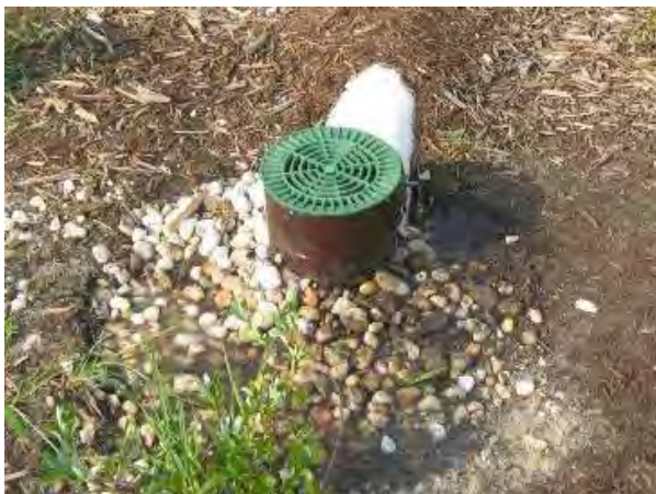
Figure A.11-4. Upturned elbow energy dissipater
