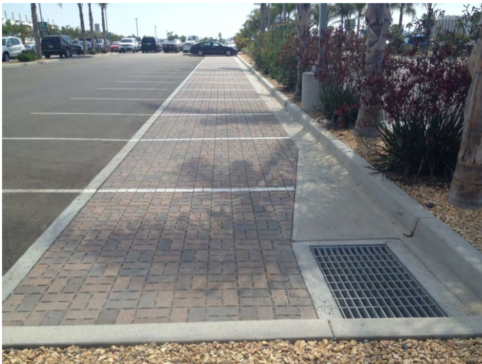
Figure 4-26. Surface overflow was provided for larger storm routing. Generally, internal bypass is effective for PICP applications to prevent upwelling and transport of the bedding course materials, but gradual slopes and diffuse flows deemed internal bypass unnecessary for this site.
