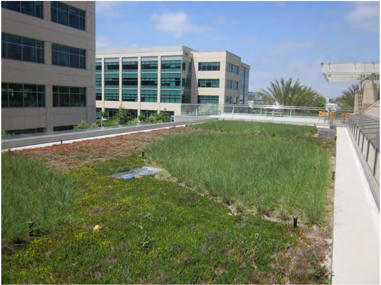
Figure A.6-1. Vegetated (green) roof.
