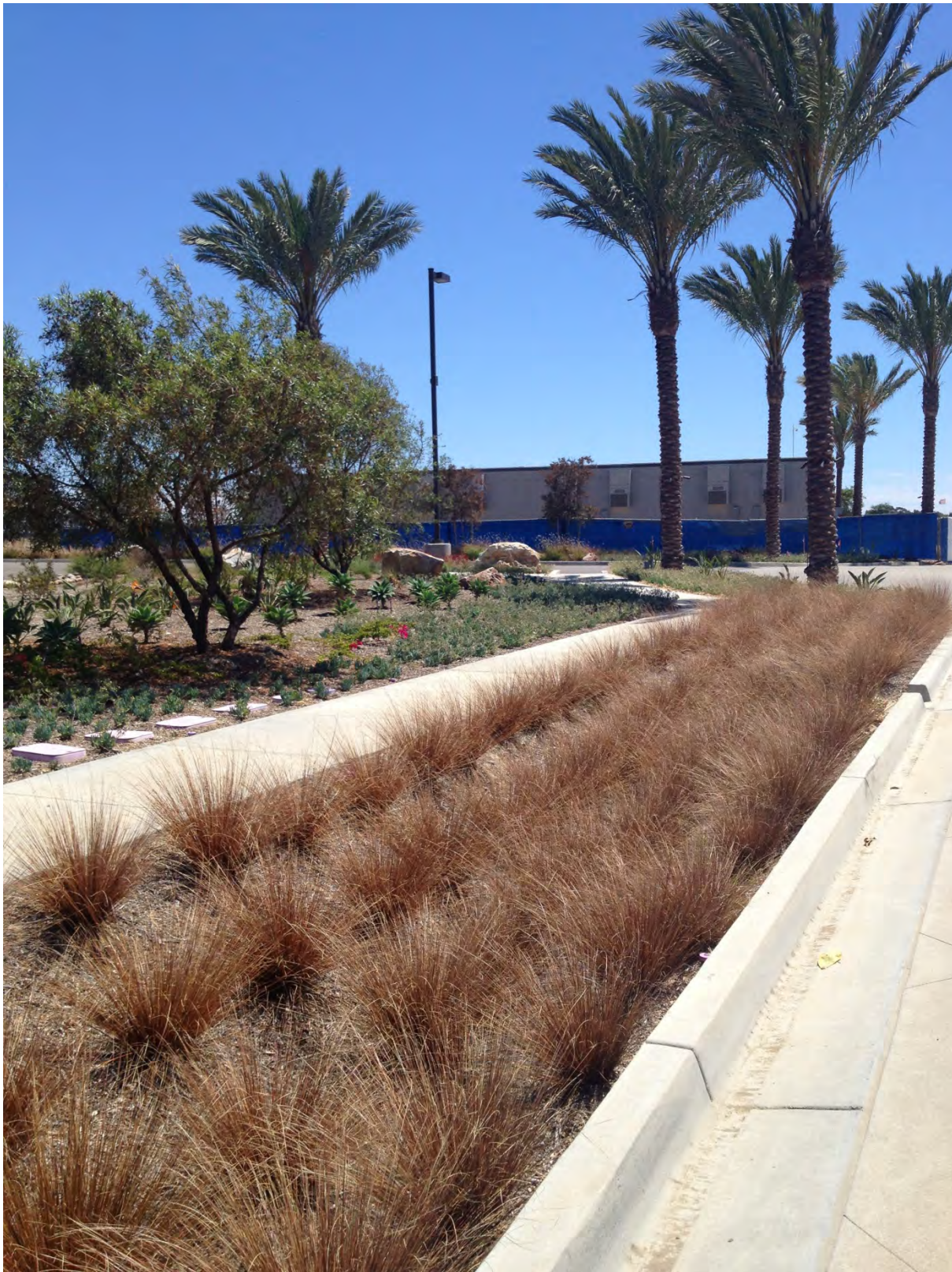
Figure 4-30. Curb cuts accept gutter flow from driving lanes into bioretention swales.
