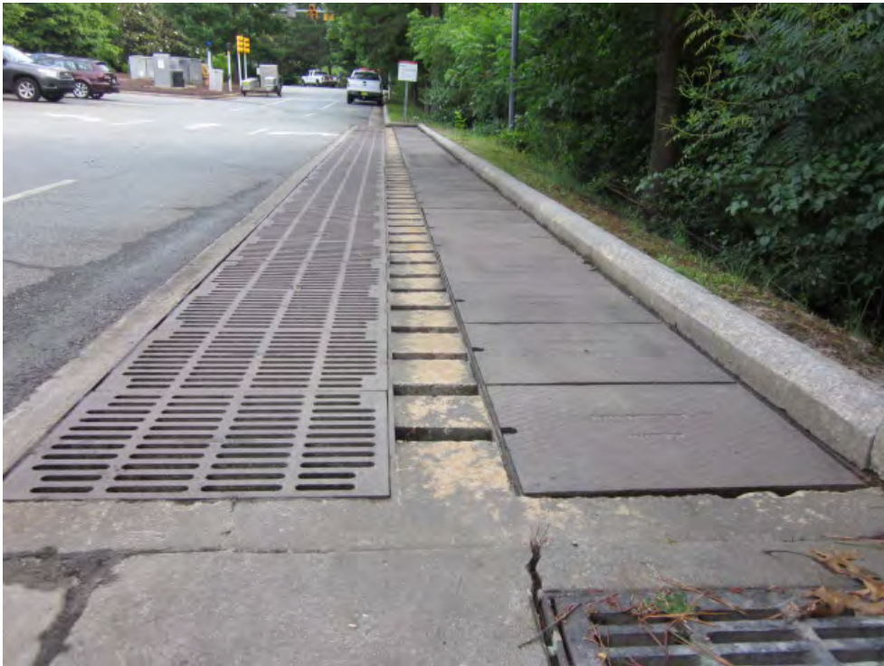
Figure 3-37. Subsurface sand filter in parking lot.
