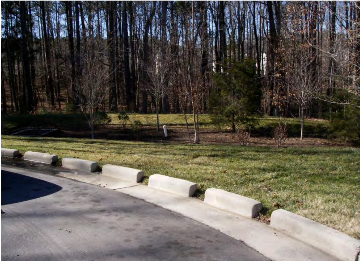
Figure 3-49. Vegetated filter strip treats roadway runoff draining to a bioretention area.
