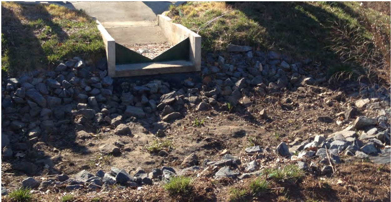
Figure 4-13. Inlet curb cut with a v-notch weir.
