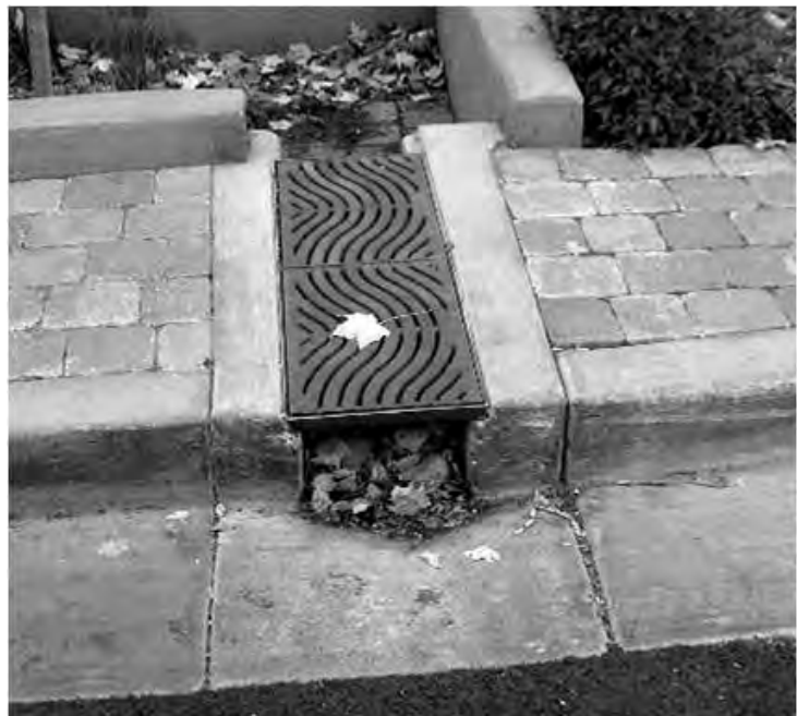
Figure 4-7. Inlet sump to remove gross solids.
