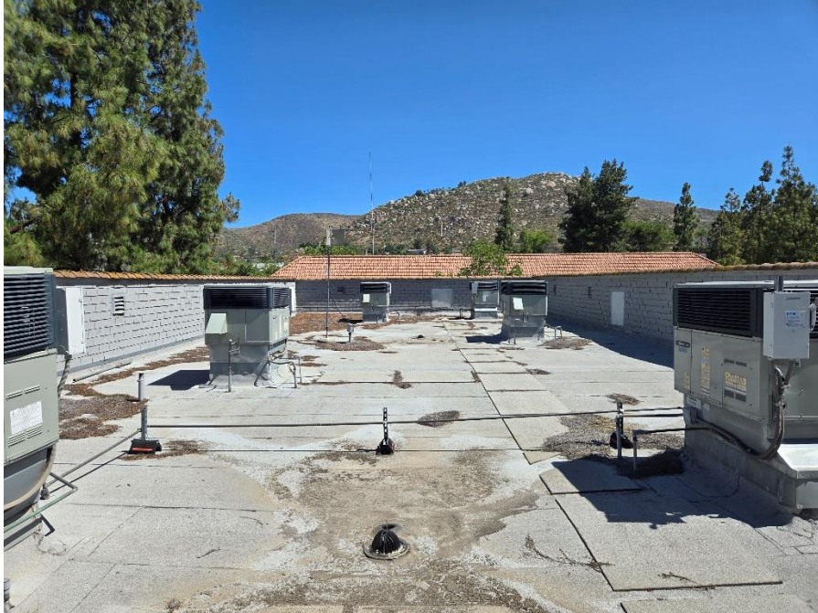
Facing North, standing at South end of roof
