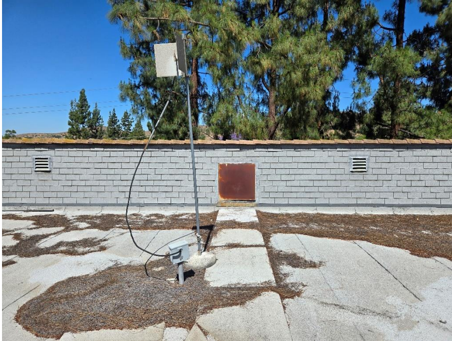
Facing West, looking at main roof attic access door
