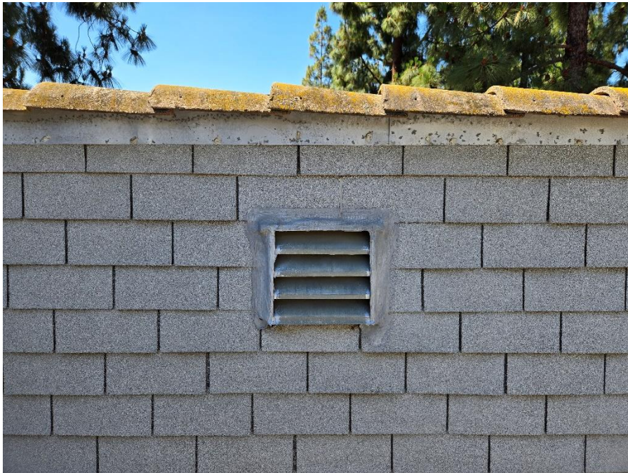
Typical Parapet Wall Vent
