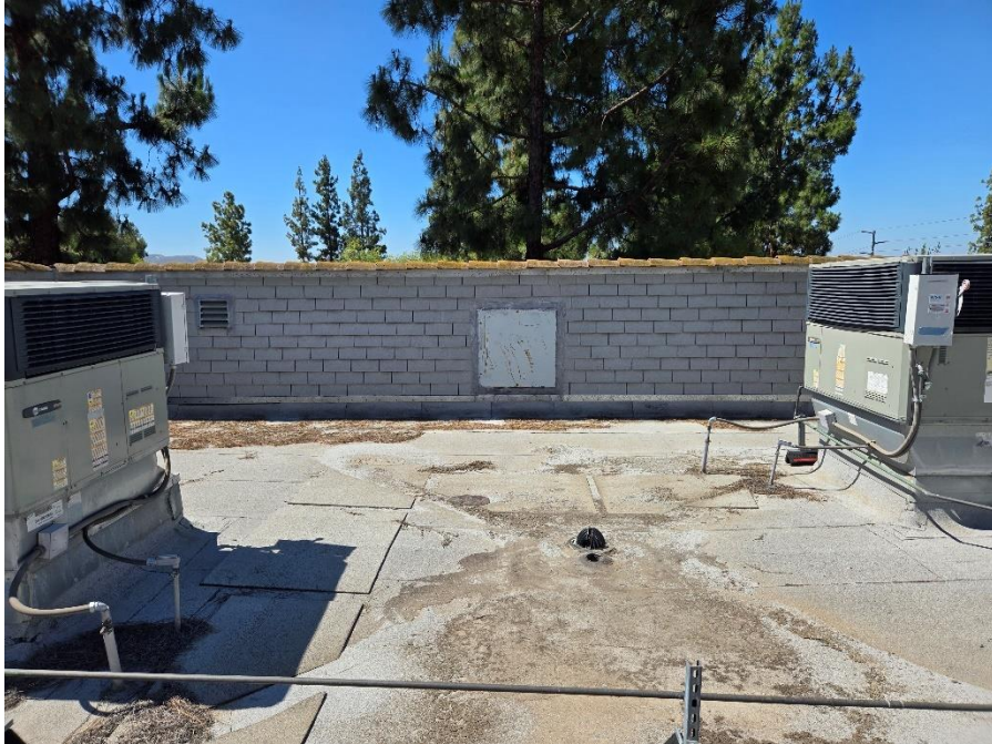
Facing South, looking at roof access door
