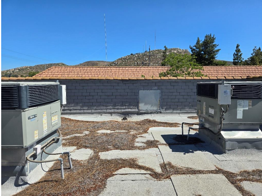
Facing North, looking at roof access door
