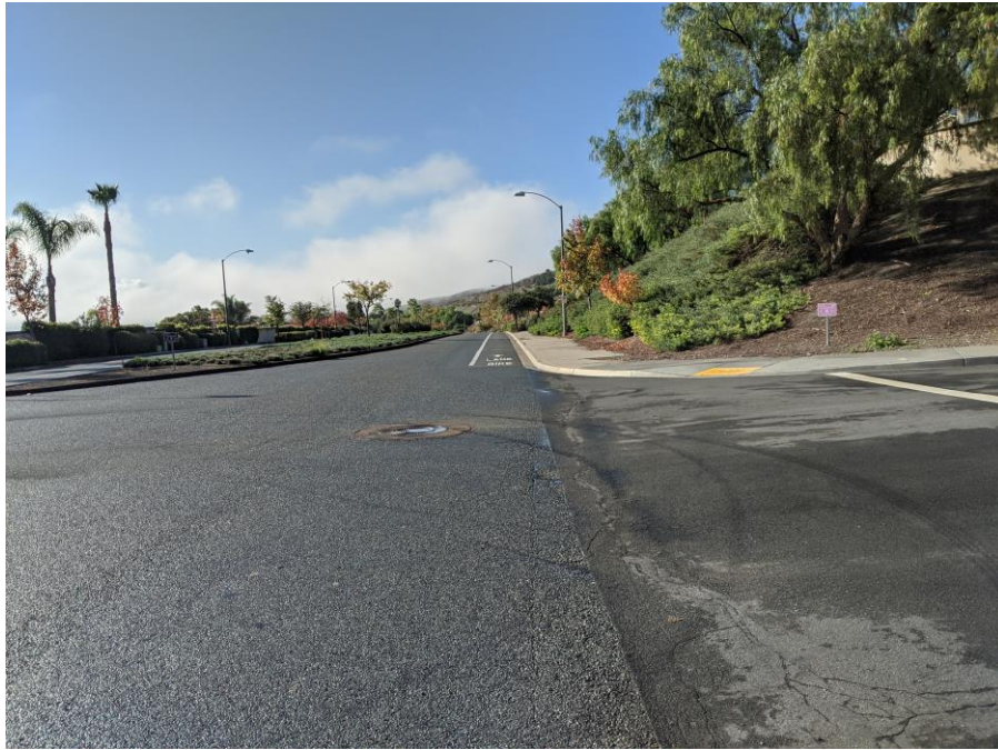
Photograph #9 Existing Cuyamaca Street in the southeastern portion of the Site.
