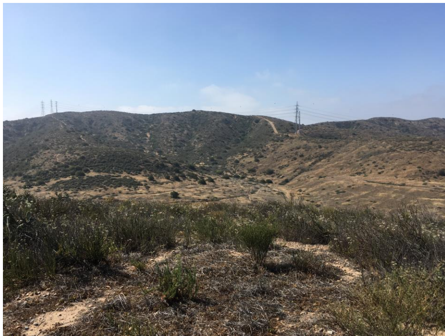
Photograph #6 View to the south of southern portion of the Site and overhead power lines.
