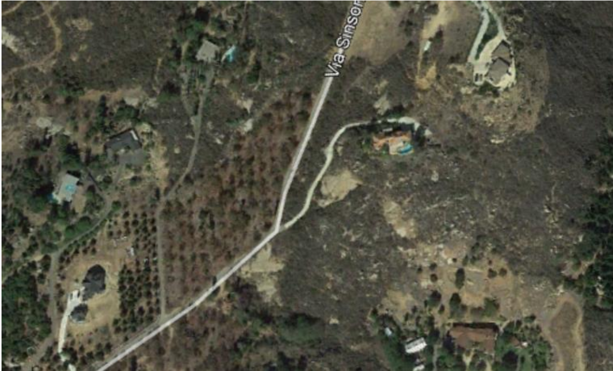
Figure 8. Example of “lower density” development where homes are interspersed amongst wildland fuels, are of varying ages, and include varying levels of fuel modification zone setbacks. Homes are exposed on most or all sides by flammable vegetation and properties rely solely on owners for maintenance, are often far distances from the nearest fire station, and have minimal buffer from on-site fire spreading to wildlands.
