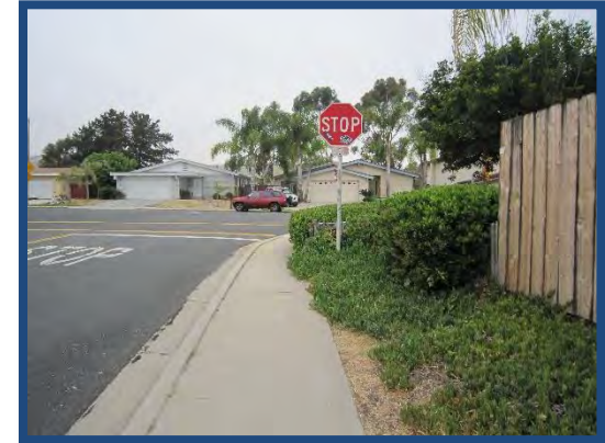
FIGURE 21 - WETHERSFIELD AND RUMSON OVERGROWN HEDGE
