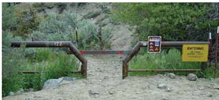
Figure 18 -- Motorized Vehicle Exclusion Gate
