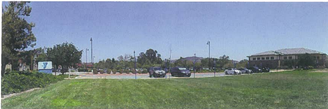
Main entrance road, looking east
