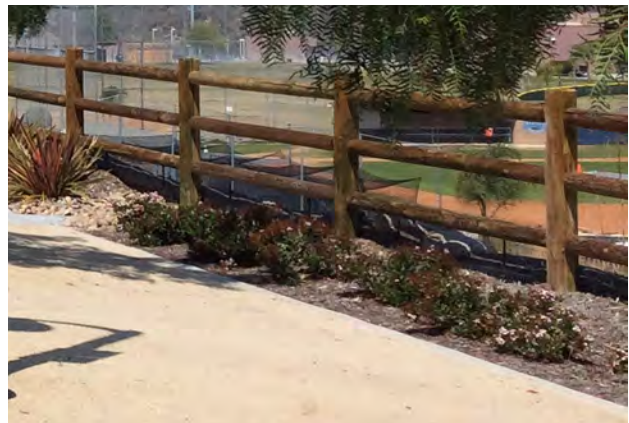
Post and Rail Trail Fencing
