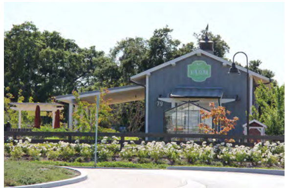
Examples of community buildings, including a clubhouse and a farm activity center.
