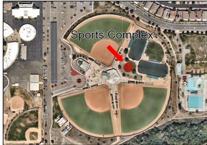
Project Location: SportsPlex at Town Center Community Park
