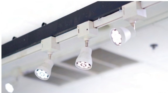
Exterior Lighting is Installed to Enhance Safety Around the Area
