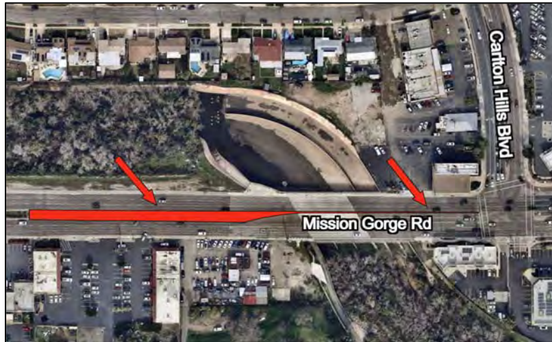
Project Location: Mission Gorge Road, Fanita Drive to Carlton Hills Boulevard.
