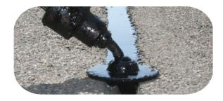
Occasionally, crack seal may not be applied to cul-de-sacs, patching areas or within 4' of a concrete gutter if the street is scheduled for an overlay or patching. The edges of the street are ground as part of the overlay process which would remove portions of the crack seal material. Omitting these areas of crack seal will save material and also reduce the cost of the project.
