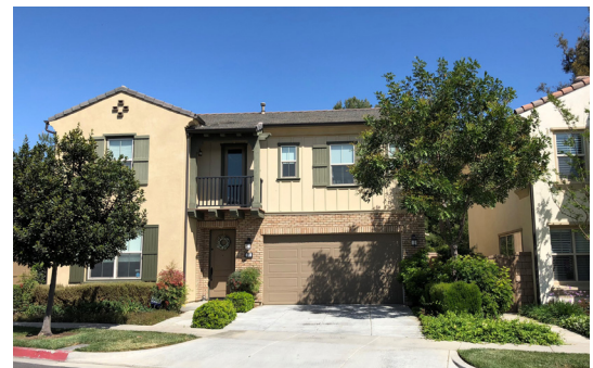
Z-Lot Homes are designed to sit together along a shared lot line by providing one home with a deeply recessed garage. Reciprocal use easements are provided to maximize side yard areas.
