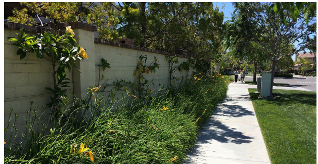
Masonry Community Wall
