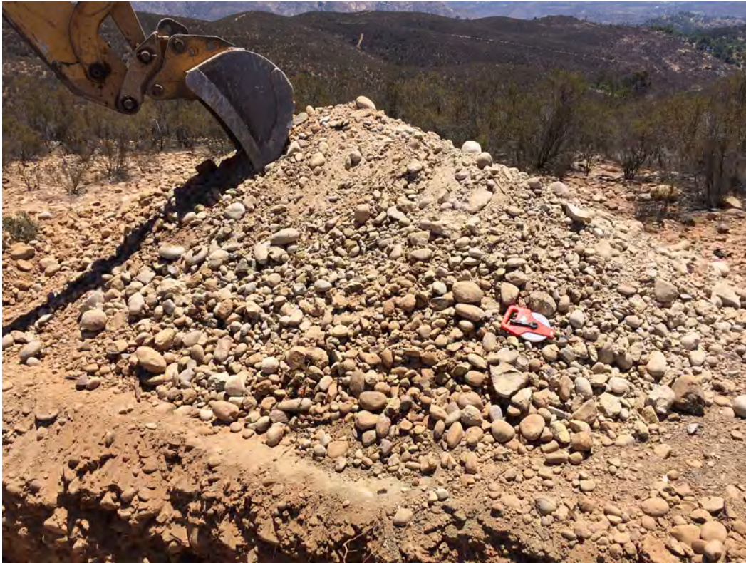
Photo 2 - 31 Trench T2 Stockpile
