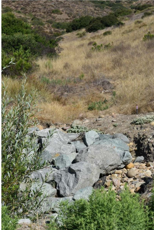
Natural rocks meet the boulders brought in by development to manage a stream the flows during the rainy season.
