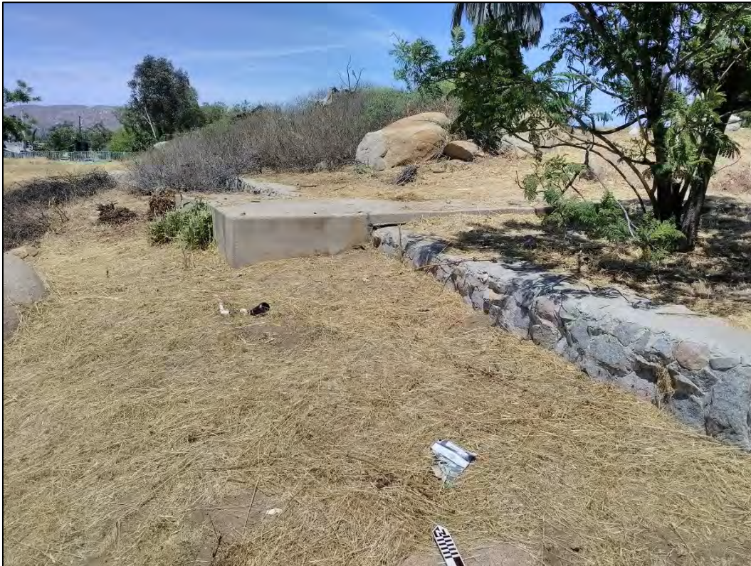
Figure 10 Feature 18, View North
