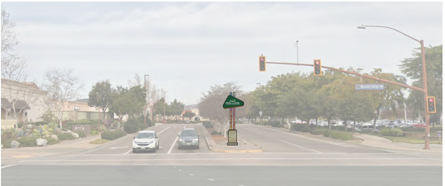
Figure 3-40: Median Identification Monument - Mission Gorge Road and Riverview Parkway
