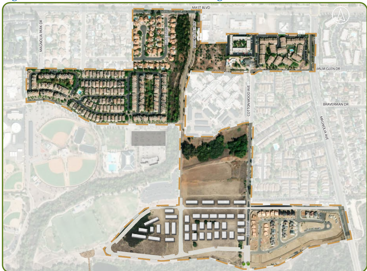
Figure 2-17: Mast Boulevard Residential Neighborhood
